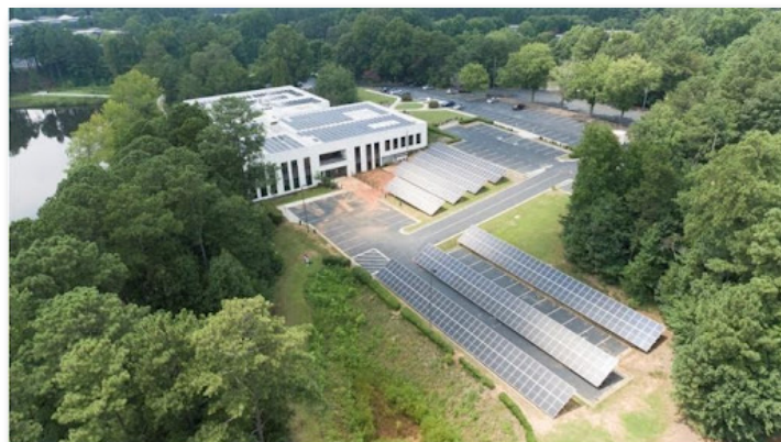
ASHRAE's recently installed photovoltaic (PV) system.
