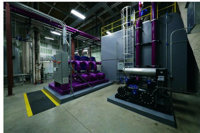
The recycled water system supplies all toilets, urinals and irrigation. The skid is a four-stage pump system
